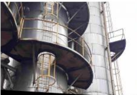
H/D Plant Tower Loading Foundation Project
