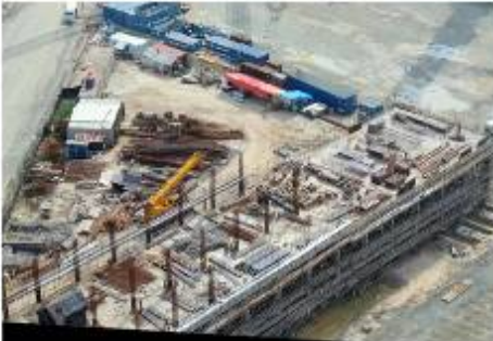
RDMP RU-V Balikpapan Building Work Package 1 Project
