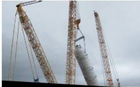
RDMP RU-V Balikpapan Steel Structure & Mechanical Work Package 1 Project
