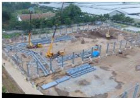
RJ3 New Building Construction Project
